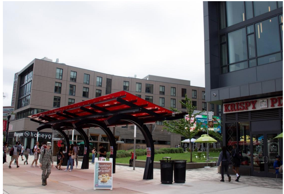
Bus Shelter at the Yard – New Brunswick
